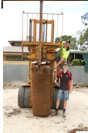
Carport removal Todd Street November 2013
